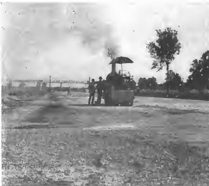
Rolling Crushed Stone on Top of Old Track Surface
